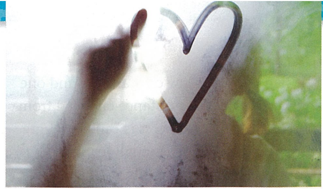
Condensation on a window
